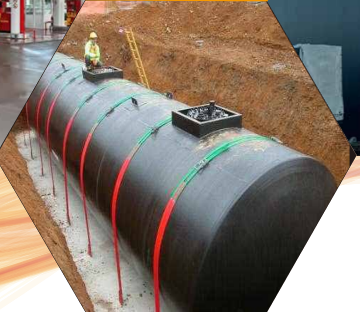
Preparing and Installing Fuel Tanks
