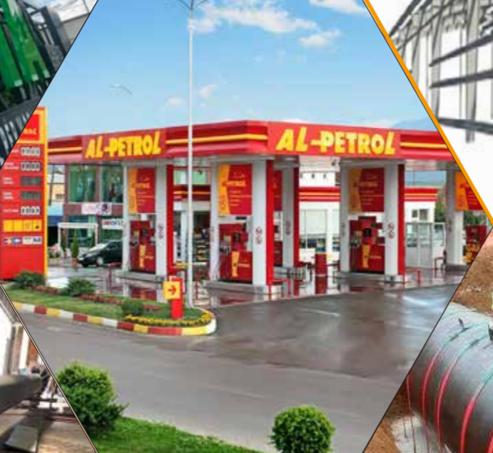
Building Oil Stations
